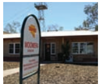
Outside photograph of the newly refurbished Woomera CFS Station which includes a kitchen, offices, meeting room and toilets.
