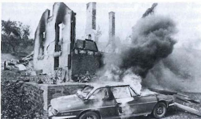
A National Trust-registered home at Paechtown was reduced to a shell by the fire. (Photograph reproduced courtesy "The Advertiser")
