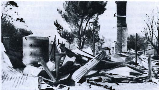
The remains of a house near Cudlee Creek. (Photograph courtesy "The Bunyip", Gawler).
