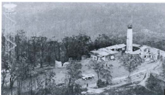
The new National Parks and Wildlife Services Fire Tower (left) and Mount Lofty obelisk survived the fires — but surrounding buildings (restaurant and facilities) were destroyed. (Photograph reproduced courtesy "The News and Sunday Mail")
