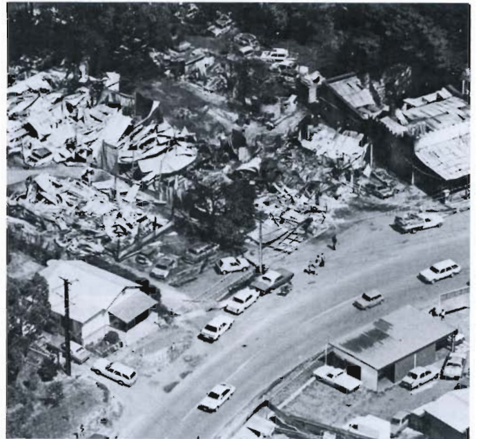
Aerial view of destruction. (Photograph reproduced courtesy "The Advertiser").
