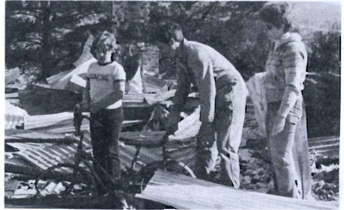
C.F.S. volunteer Chris and Lynda Osborne's home was among 7 destroyed in Cudlee Creek. Sadly destruction was so severe that even daughter Lynda's bicycle was not worth salvaging. (Photograph supplied courtesy "The Courier", Mt. Barker)
