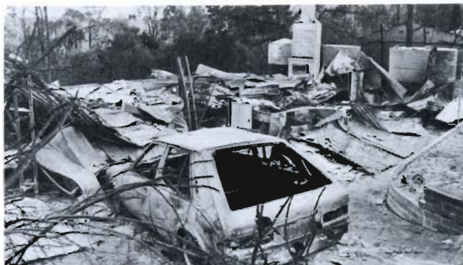
One of the houses destroyed in Yarrabee Road, Greenhill. (Photograph reproduced courtesy "The Advertiser").
