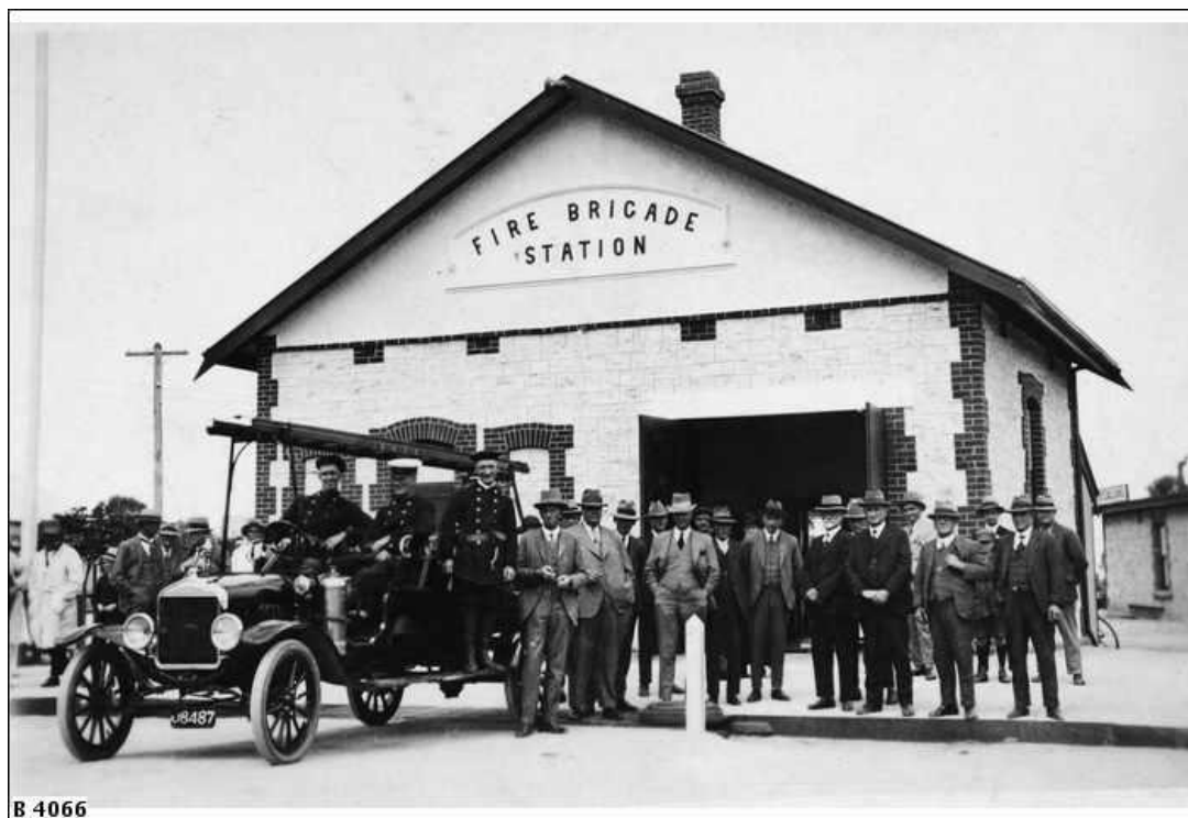
State Library of South Australia - Image B4066.jpg, Fire Brigade Station, Balaklava. The new Fire Brigade Station remodelled from the old Council Chambers. Opened by the Chairman of the District Council Mr. W. Manley, 15 March 1927 - the Fire Brigade Officials in the foreground. 1927
